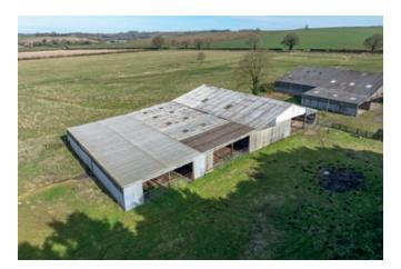
**3.** Open Fronted Machinery Store (968 ft² or 90 m²) 4-bay, timber framed with profile steel sheet cladding to mono-pitch roof and sides. Compacted floor.
